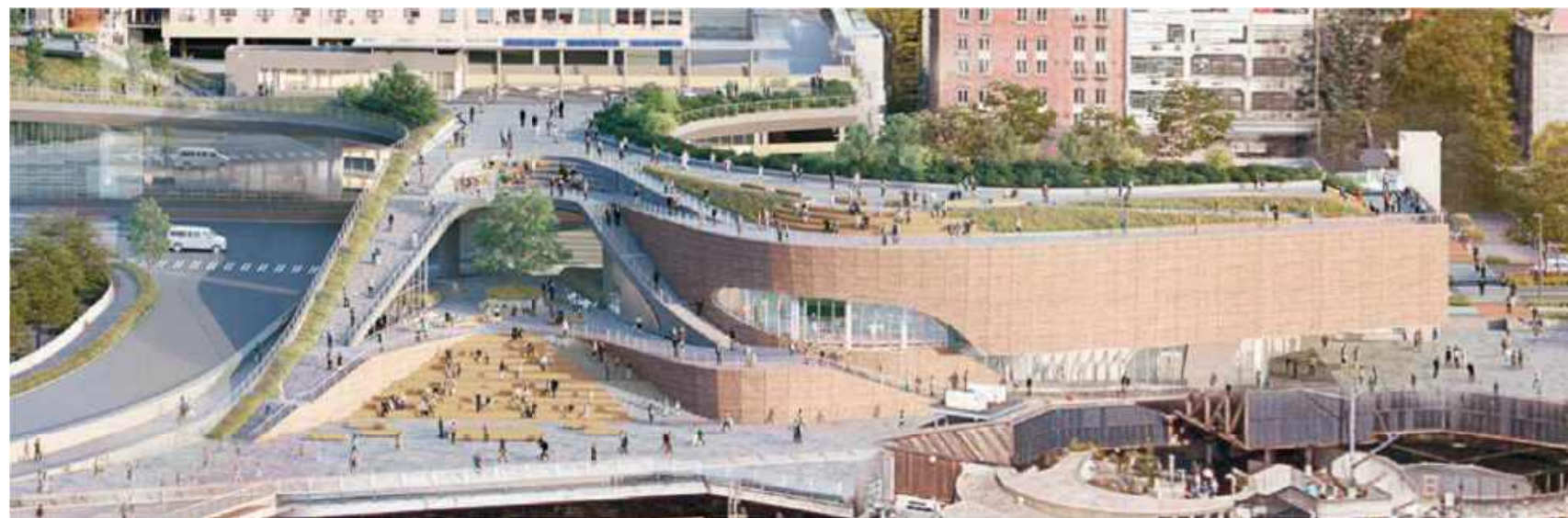
West facade of Ocean Pavillion
