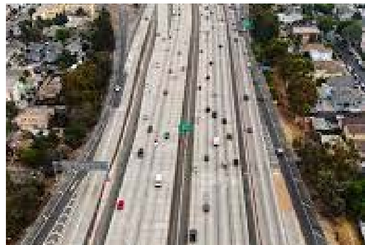
I-10 Freeway is a major generator of noise in proximity to the site.
