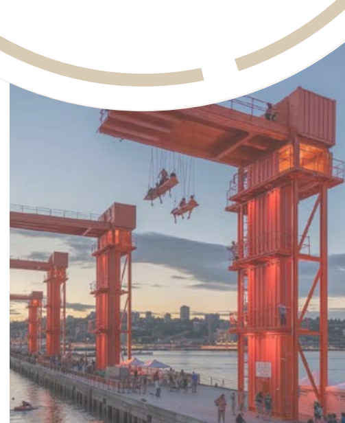
Angular trellises and towering frames create a bold, directional rhythm.
