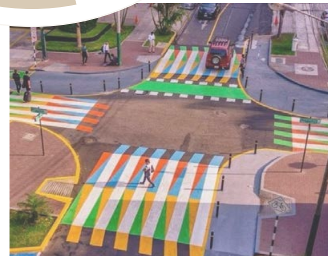
A vibrant crosswalk that doubles as a traffic-calming device—inviting drivers to slow down, signaling that something worth noticing is just ahead.
