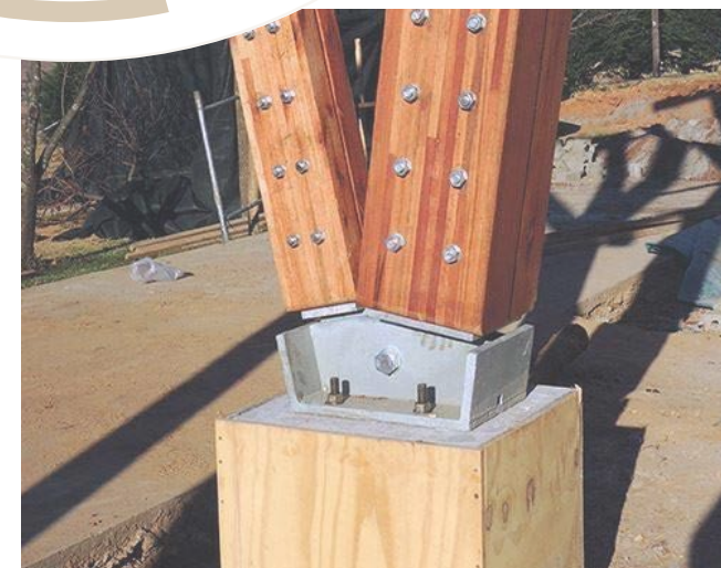
Truss and joiner form
