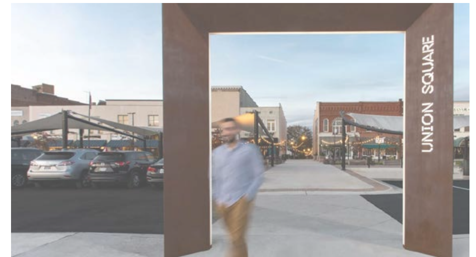
Blending of portal structures with signage, framing the space and inviting user experience
