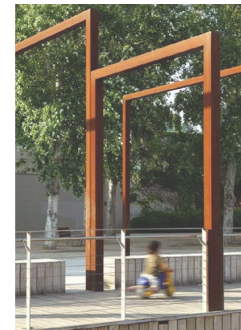
Portal structures offset. Corten steel and reclaimed wood.
