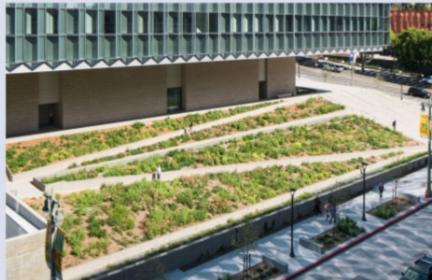
Los Angeles Federal Courthouse - Studio-MLA
