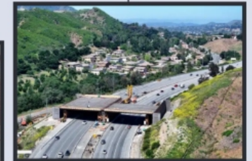
Wallis Annenberg Wildlife Crossing under construction
