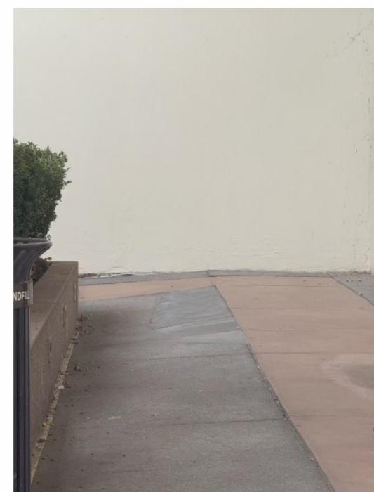
WATER DRAINAGE SLOPE
