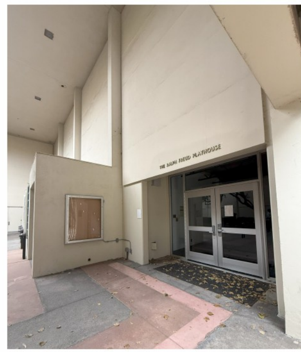
THE CONSTRUCTION OF THE VESTIBULE
