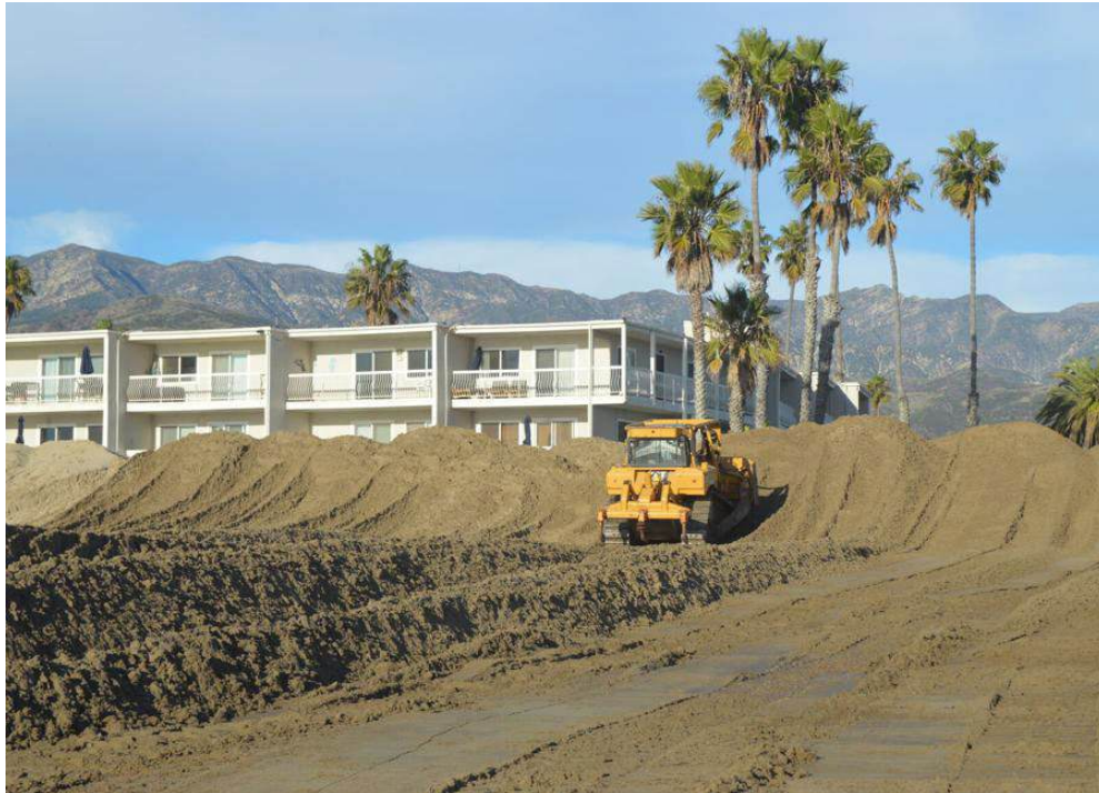
WINTER STORM BERM BEING CONSTRUCTED
