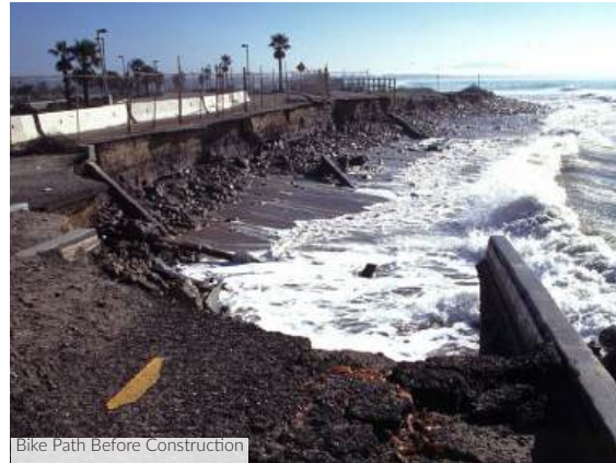
Bike Path Before Construction
