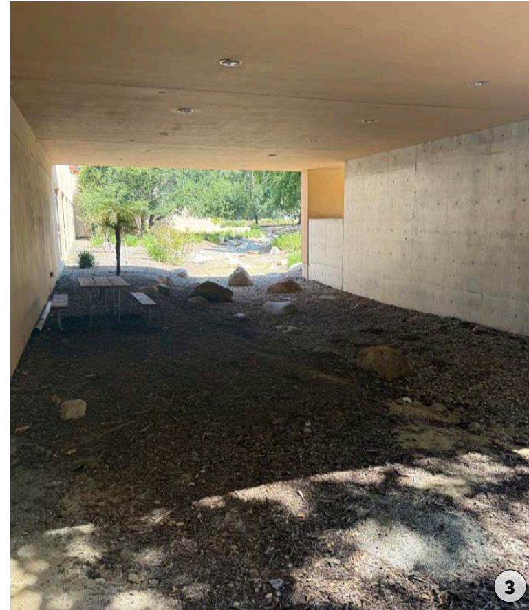
Breezeway with dry creek bed connecting zones 2 and 3
