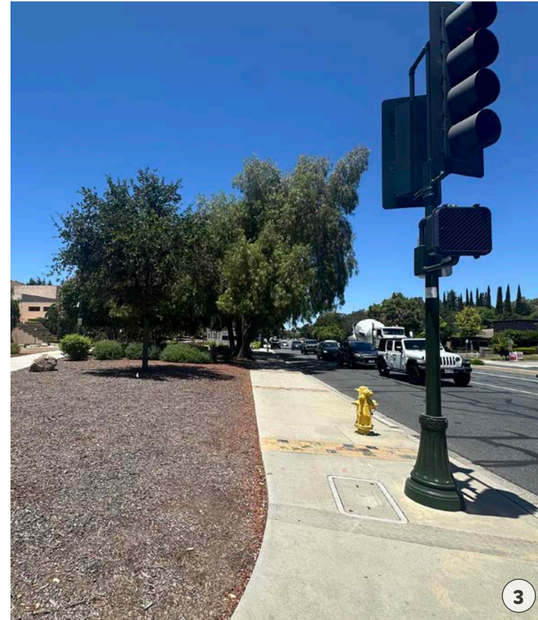
Sidewalk along Thousand Oaks Blvd near crosswalk at The Lakes Dr facing west
