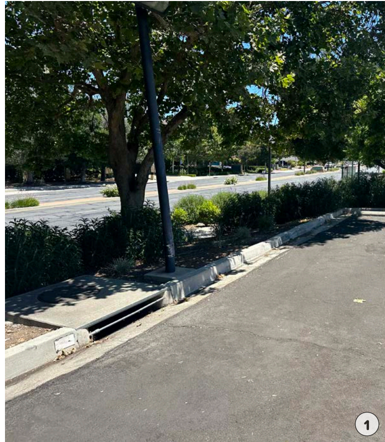
1 Northern end of the existing parking lot (to be removed) looking out toward Thousand Oaks Blvd
