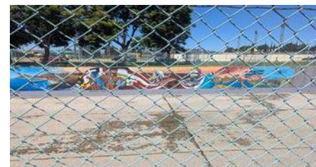
Concrete river bottom
