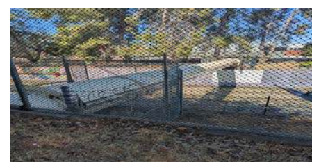
Water pipe crossing channel
