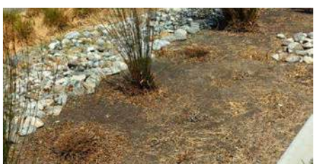
Rain garden/groundwater recharge
