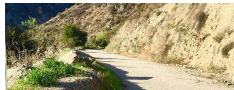
BARE GROUND ON TRAIL SYSTEM AT - AWP
