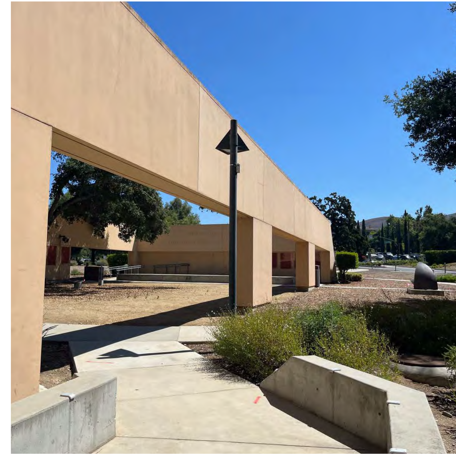
3. Exterior of outdoor stage area
