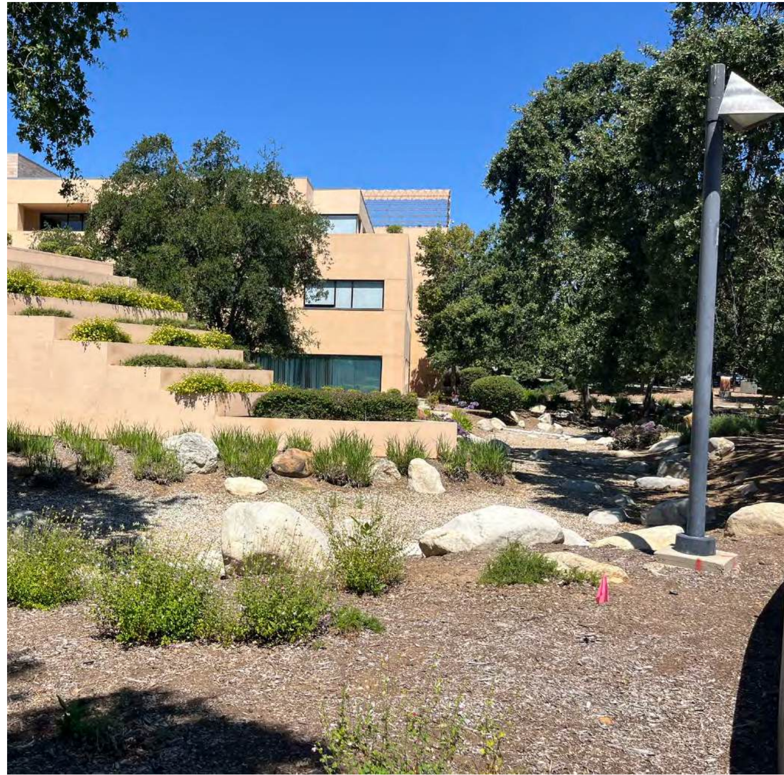
1. City Hall offices along swale
