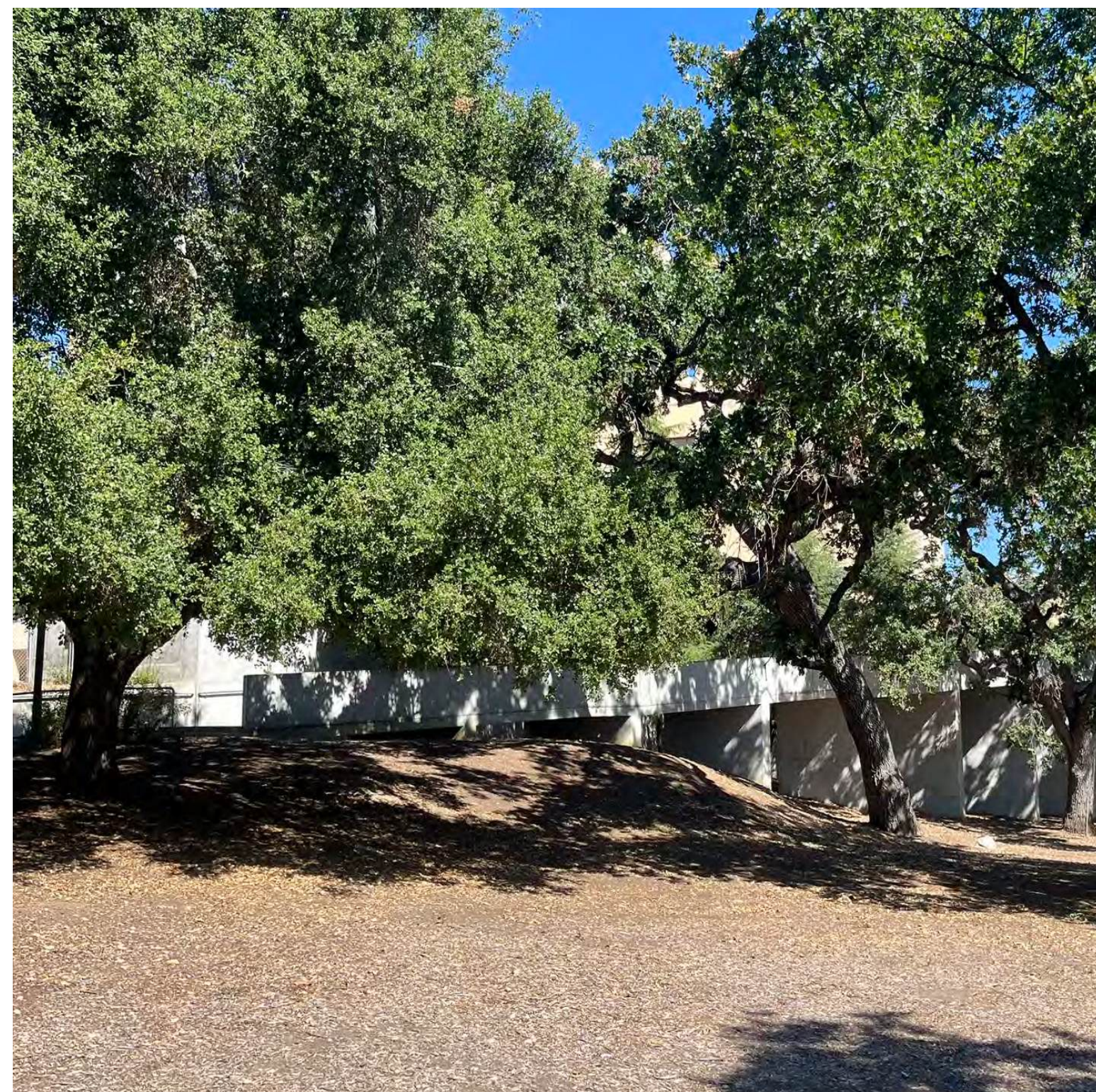
4. Ramp that connects to the second floor
