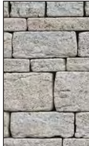
Stone Retaining Walls
