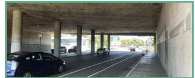
The 10 Freeway Underpass is part of the project site
