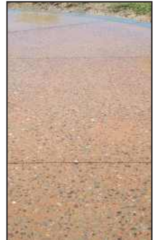
Integral Concrete Path
