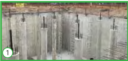
Underground Stormwater Cistern 80,000 cubic feet Subterranean Cistern
