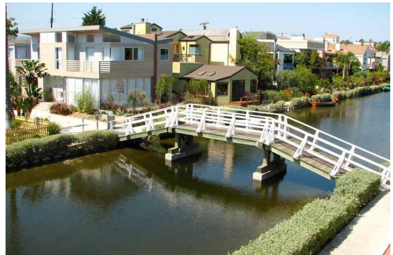
Upgraded canal with pedestrian walkways, native saltbrush landscaping and new bridge.
