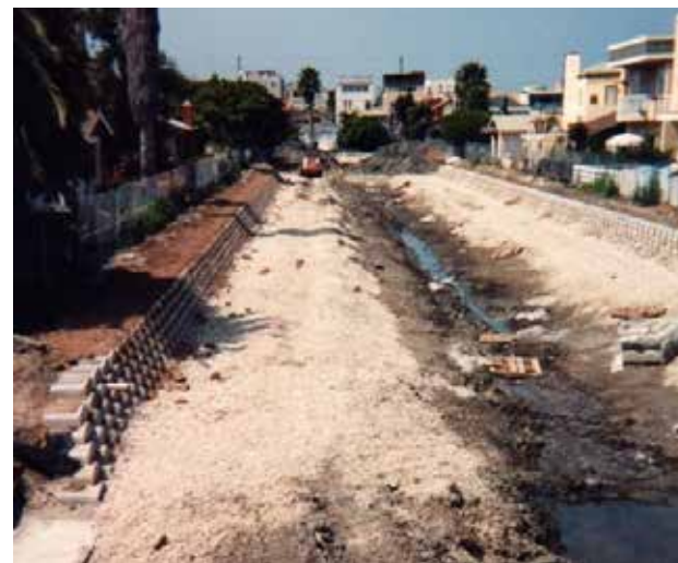
Construction for 1991-93 renovation project.
