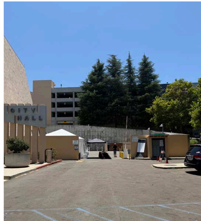
5 View to the loading dock (G). Connected to Civic Arts Plaza street.
