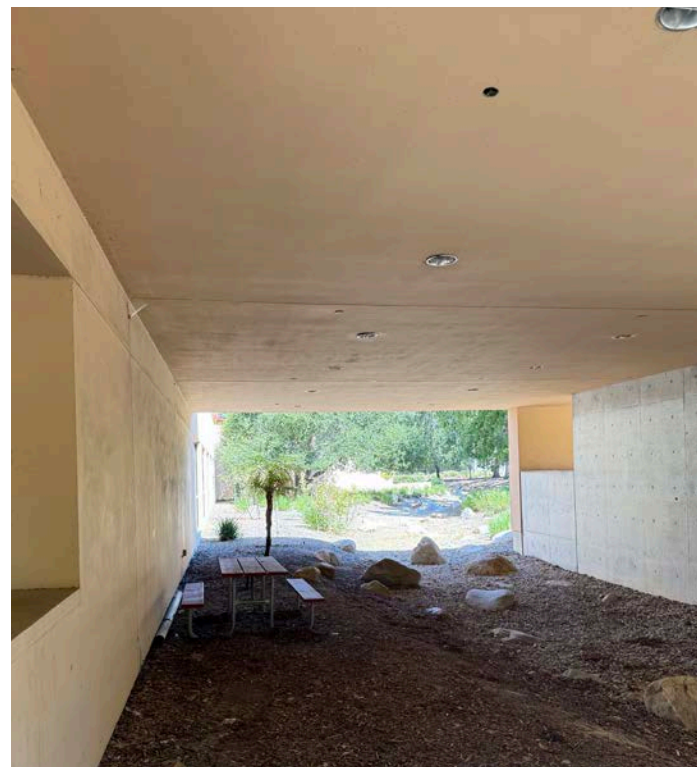
4 View of drainage swale that goes across underneath the building. Not welcoming but provides shade.
