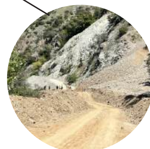
Landslide on Trail
