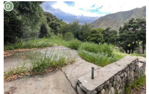
Terraced Trailer Home Parking
