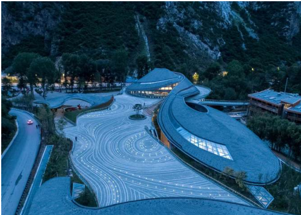
Constellation Lighting Design Integrated into Hardscape
