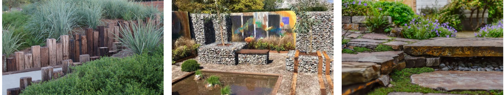
Reclaimed wood from a railroad Gabion walls for seating opportunities Stone slabs reused as pavers
