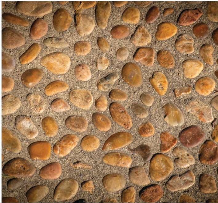
Large Aggregate Concrete Mix
