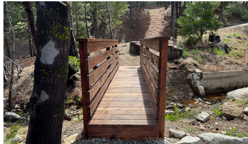
Sample footbridge that blends effortlessly into the landscape.
