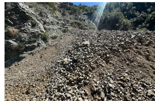
Remains of landslide on Old San Gabriel Road
