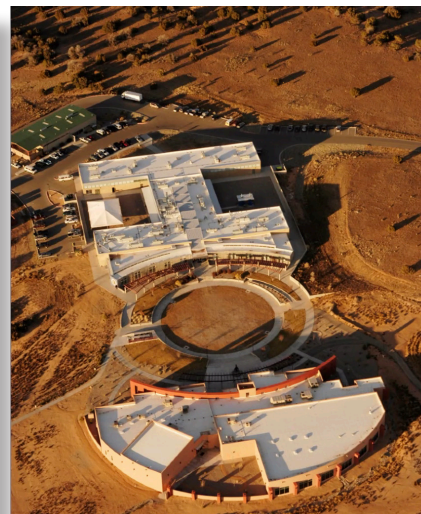
Aerial view of first phase of construction showing central plaza Photo Courtesy by Paul Fragua
