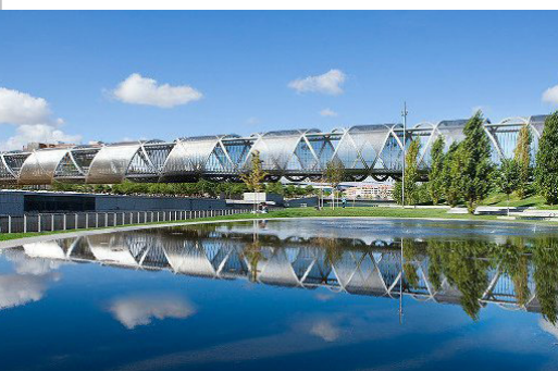
Arganzuela pedestrian bridge
