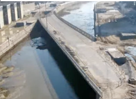
Oblique bridge before construction
