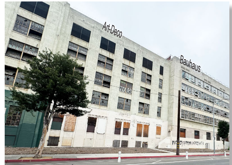
View of the Lincoln Heights Jail from Avenue 19
