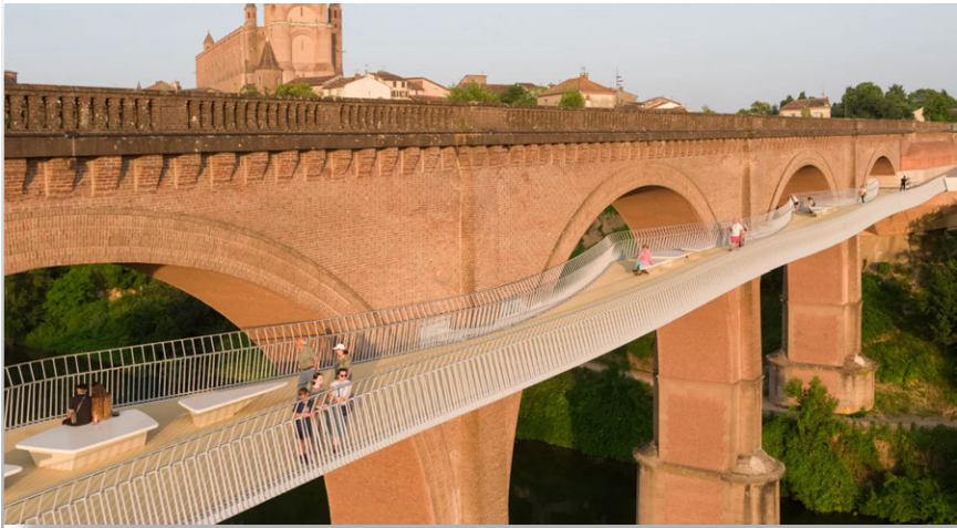
Pont Vieux d'Albi in France: a new bike and pedestrian crossing attached to an old train viaduct in Albi, France. Photo by Vincent Boutin
