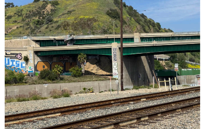
Union Pacific cargo railroad at the north end of site and 110 Freeway
