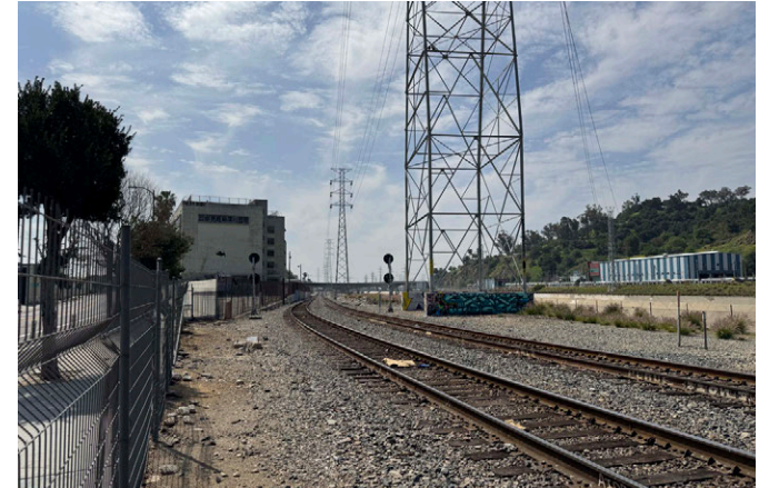
Southern Pacific railroad and transmission towers at north end of site
