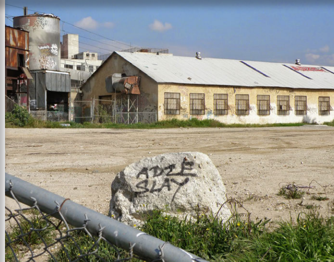
Pre-existing conditions. Photo courtesy of www.evanescentcityblog.com
