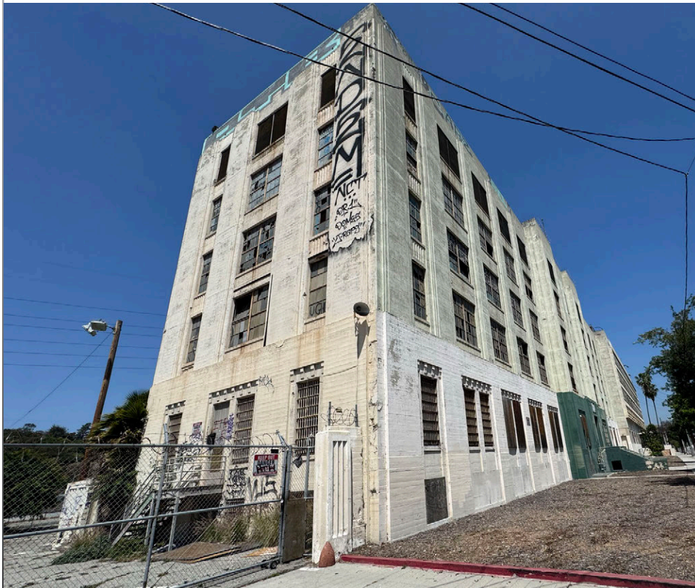
Copper wire theft has exasperated the amount of asbesot and lead that are leaching into the concrete walls, floors, ceiling and basement of the jail.
