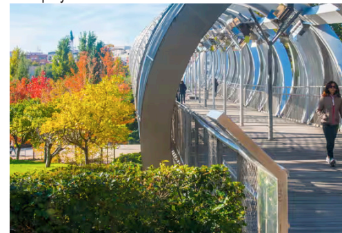
Arganzuela footbridge over the Manzanares River
