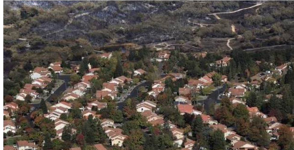
FOOTHILL REGIONAL PARK AND TOWN OF WINDSOR POST 2019 KINCADE FIRE
