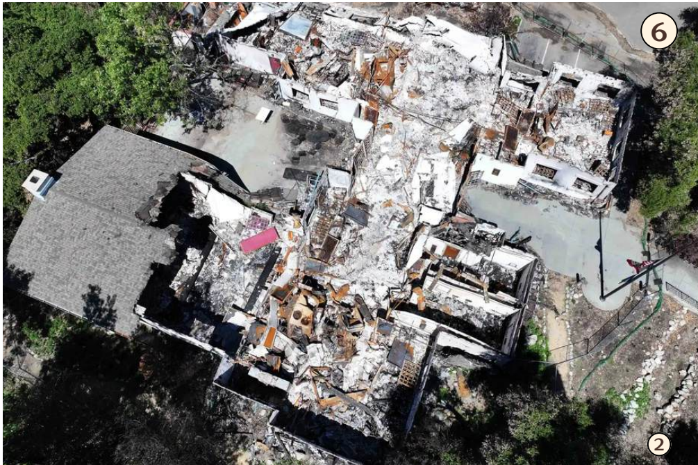
OVERHEAD OF NATURE CENTER DAMAGE
