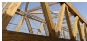
Wooden bridge with metal mesh
