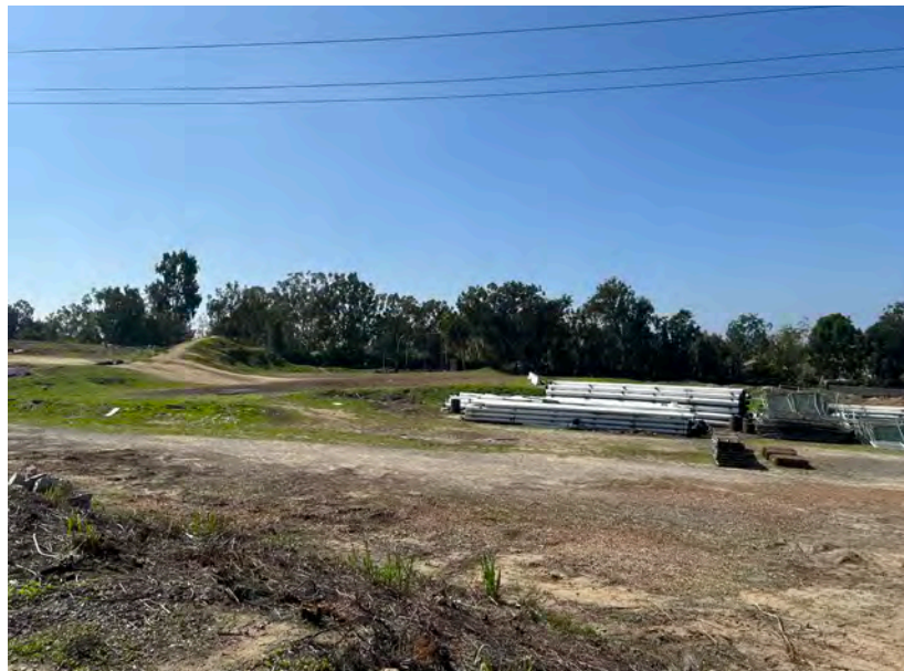
5. Looking south at industrial material waste on site
