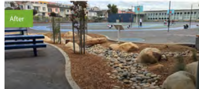
Bioswales are cut into hardscape to manage stormwater runoff 1
