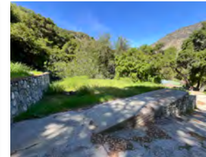
(F) STEEP FORMER RV PAD AREA
