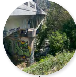
POTENTIAL CONNECTIVITY TO MULTI-MODAL TRAIL UNDER BRIDGE IS VERY STEEP
