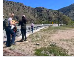
(C) BRIDGE UNSAFE FOR CROSSING
