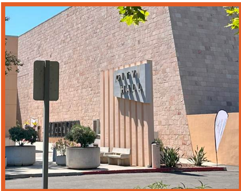
4 Square columns used at two main signs.
