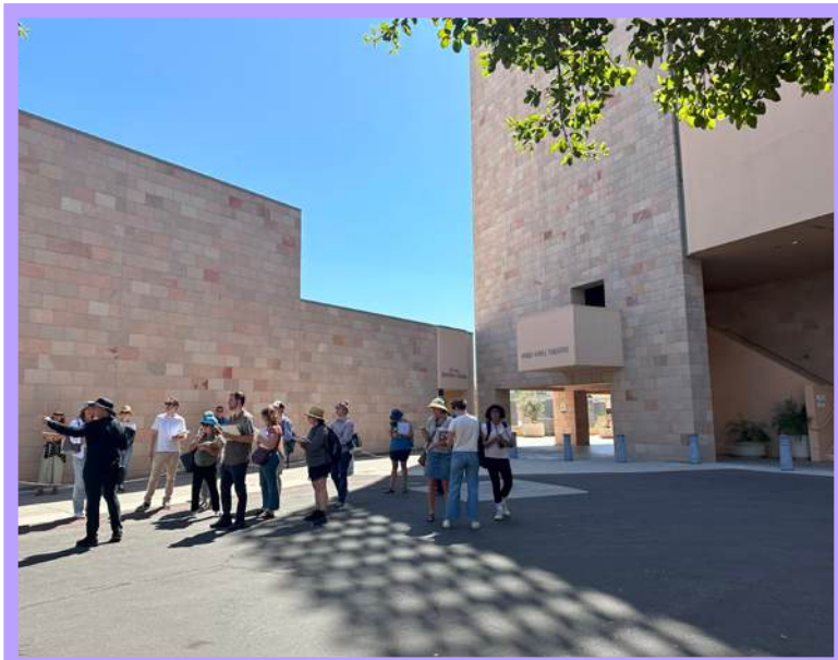
4 Entrance to 3rd floor terrace (+28) and Kavli Theater from circular car drop off.
