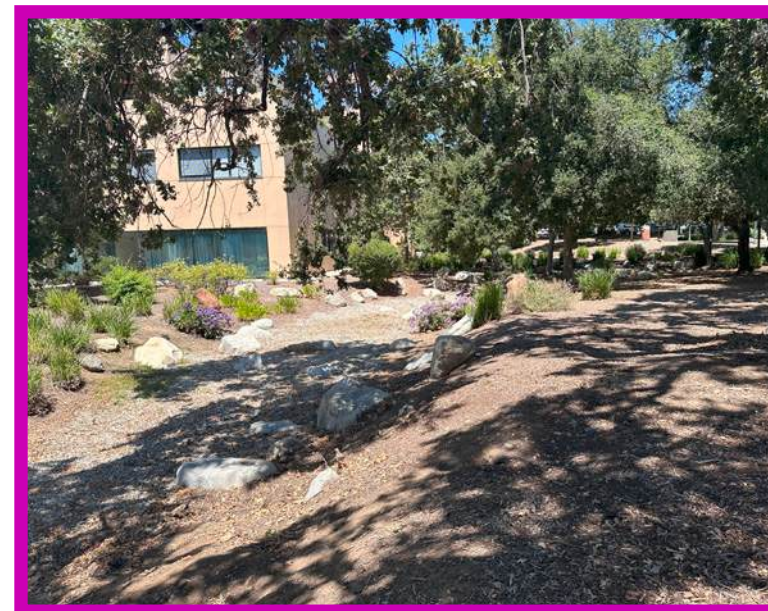
3 Drainage swale along front of building. Facing Zone 1, with theoretical City Hall entrance on left. Note shady Oak grove.
