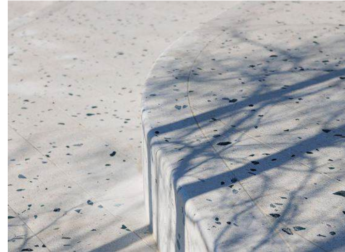
Terrazzo Aggregate Concrete
