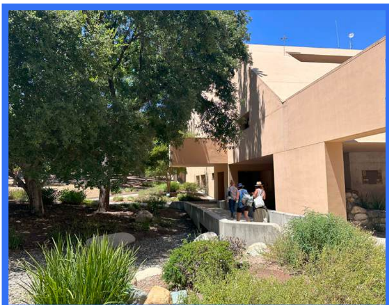
4 Secondary side building entrance underneath cantilevered 2nd floor balcony, accessed via pedestrian bridge over drainage swale.
