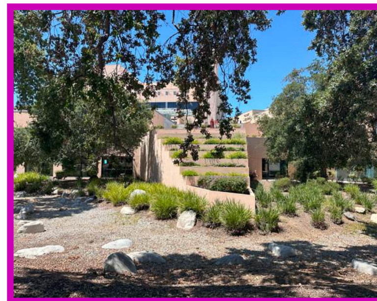
6 Continuation of architectural terraced stairs at ground level, used as planting terraces. Hidden from view by Oaks in foreground.
