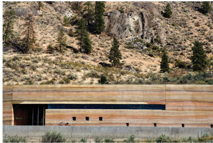
Rammed earth for new buildings is a great way to connect to the nuances of place and create structures that are low impact and comprised of place
