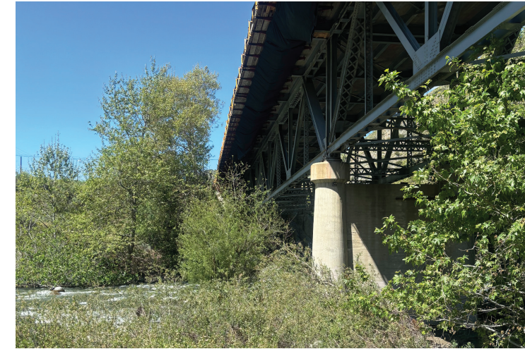
Area below highway bridge offers unique area for activation / shade
