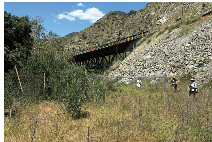
Dangerous vehicle circulation area on CA 39
