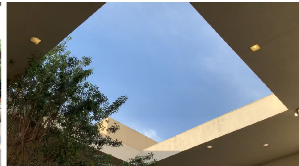
PROJECT SITE HAS A SKYLIGHT THAT IS CENTRAL TO THE COURTYARD. IT IS AN EYE CATCHING DESIGN FEATURE THAT ALLOWS SUN AND RAIN TO ENTER COURTYARD.
