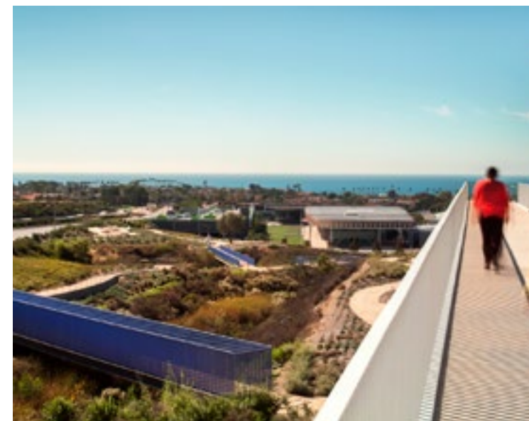
From this view point, the observer can see how the designers thoughtfully directed the site to connect with the ocean.
