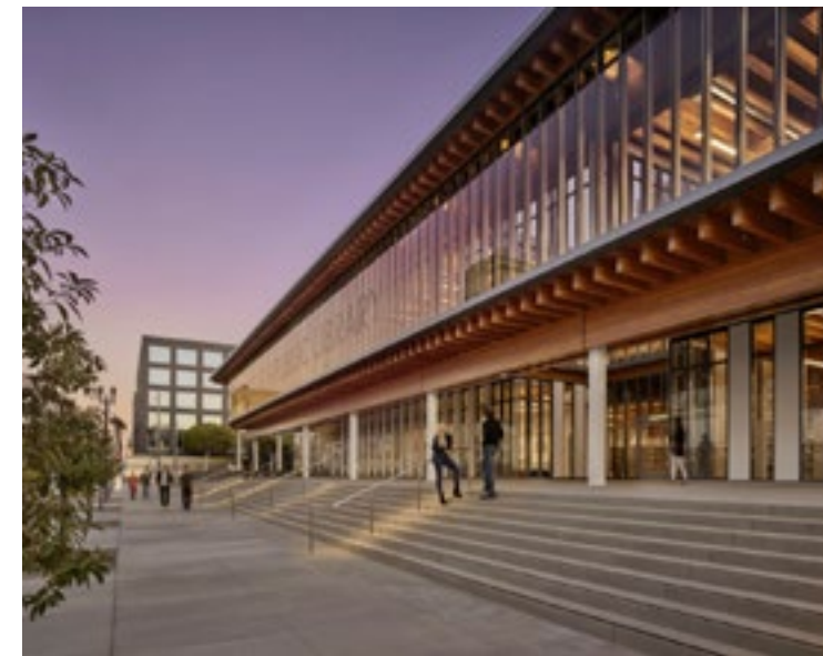
This is the north facing side of the Billie Jean King Main Library with access via secondary vehicular circulation on W Broadway.
