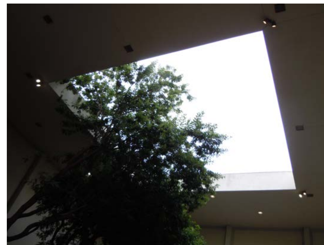
Open roof at the center of the ceiling
