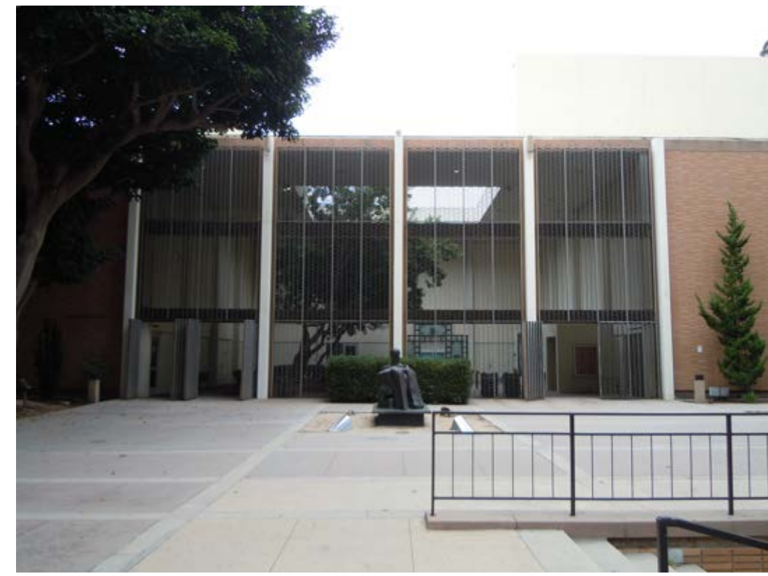
Site enclosed by galvanized metal trellis - Entrance through gates
