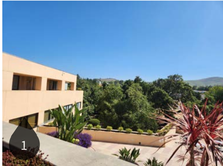
Photo 1: View from level 3 of rooftop terrace and north of site.
