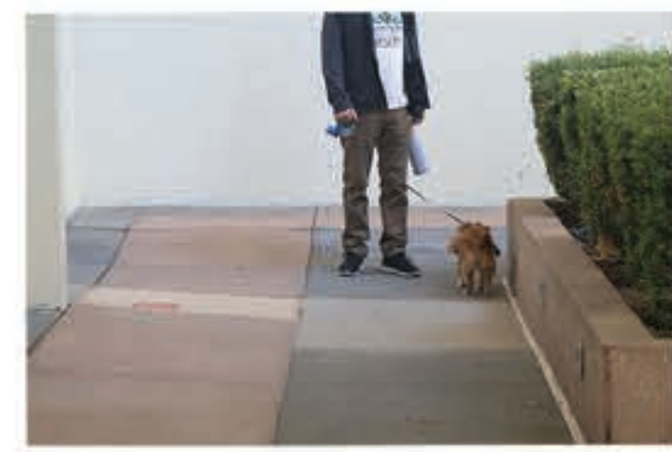
RAISED BEDS AND DRAINAGE TOO CLOSE TO WALL
