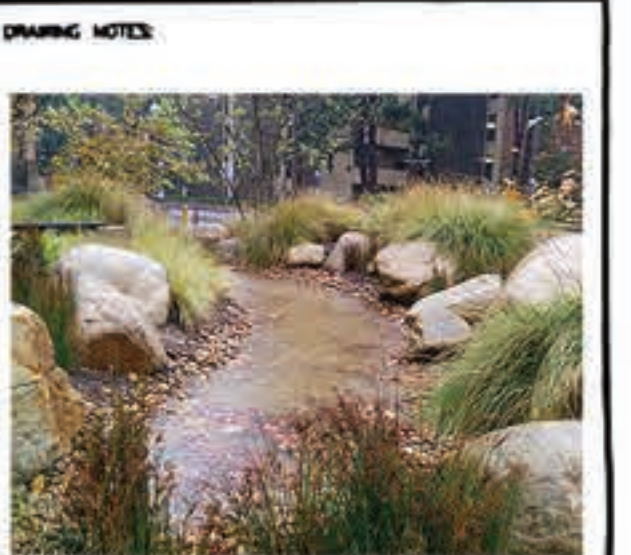
bioswale reduces runoff and foundat instability
