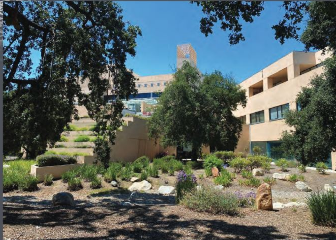
1. This stepped planter was originally designed to be a stairwell
