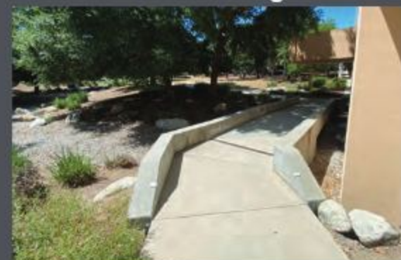
6. A small bridge over the swale
