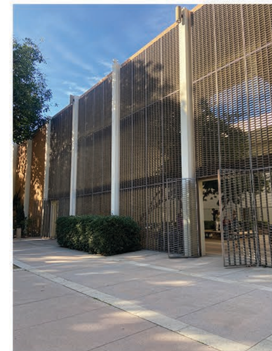
Outside view of entrances/exits
