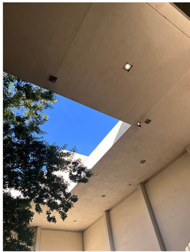
Skylight & Overhead Lighting
