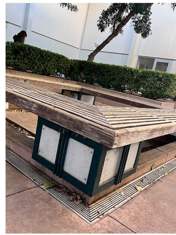
Bench, Ground Light & Drain
