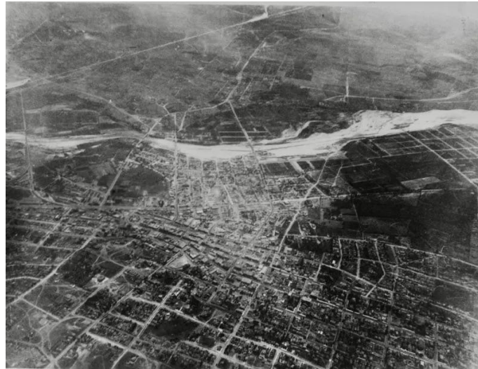
Air view of Los Angeles taken in 1887. Photo Credit: The Los Angeles Public Library Photo Collection.
