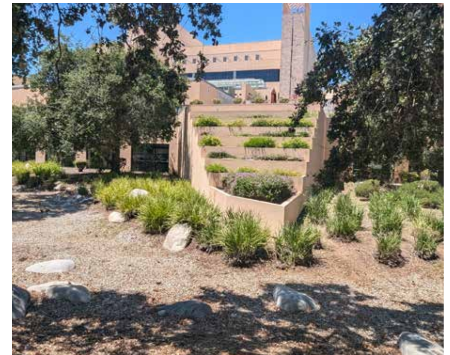
▲ LOWEST POINT OF 'SWALE' WATER COLLECTIONS DRAINS OUT TO STORM DRAIN ▲
