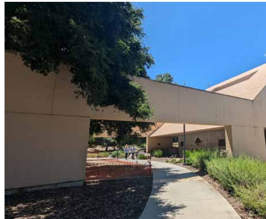
▲ FACING SE: PATHWAY THROUGH ARCHITECTURAL AMPITHEATER ▲
