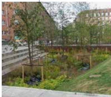
Large Vegetated Bio Swale
