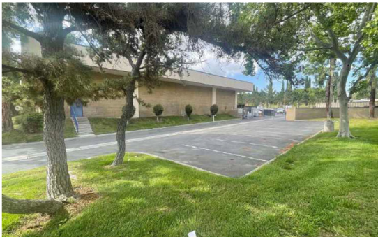
4 Riverside County Office of Education - existing parking lot.
