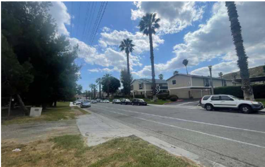
1. Lack of sidewalk along Pine Street.
