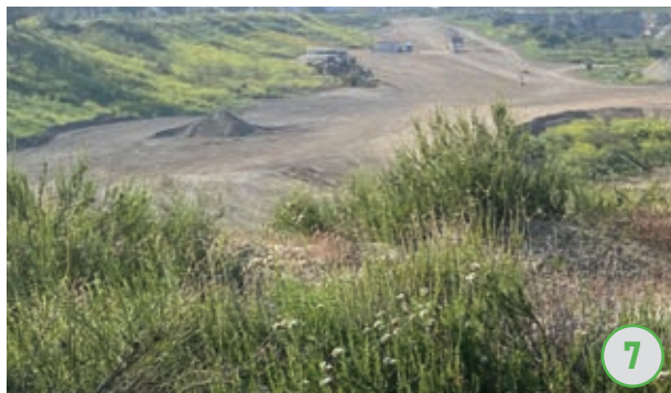
North West - Main entrance / driveway to the site
