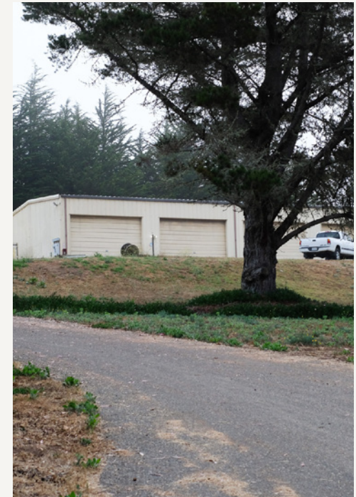
7. Existing Maintenance Shed
