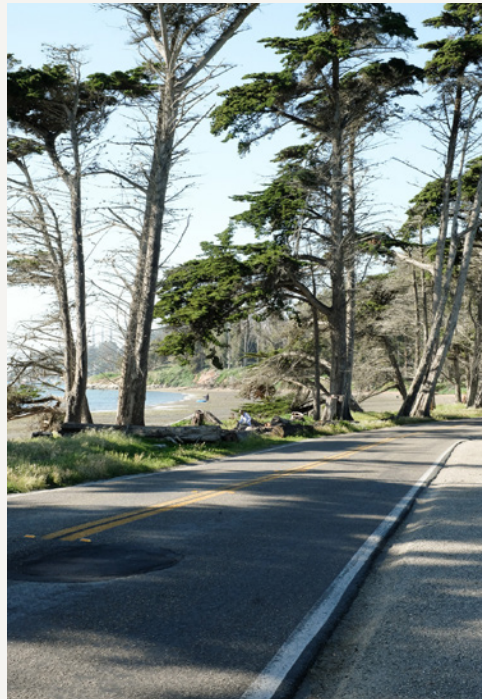
5. View of Edge Along Road
