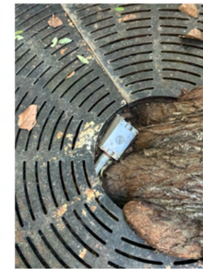
Drainage and electrical outlet.
