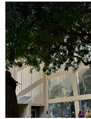
A detailed view of the grid wall revealing sunlight entering the courtyard.
