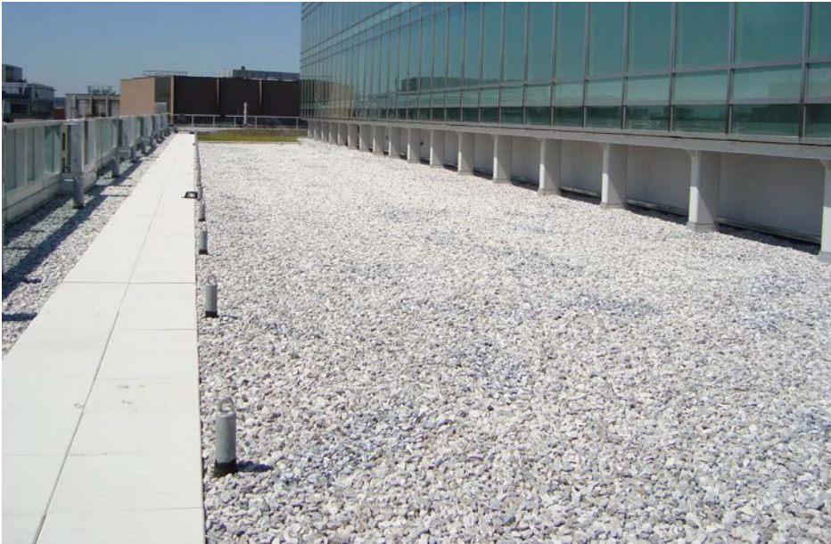
Reflective White Aggregate on Rooftops
