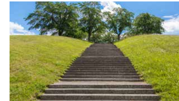
Steps to hilltop grove get less steep as you go up, so as not to tire visitors once they're at the top.
