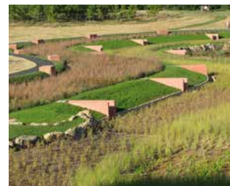
Bioretention terraced trays control overflow to wetland/pond
