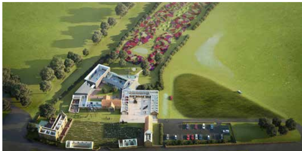
Aerial rendering during construction phase
