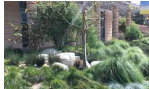
Planted swale and rain garden
