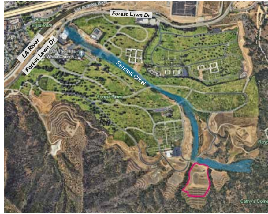
Aerial view of expansion during grading phase
