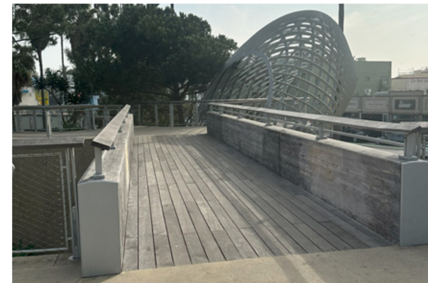
UPPER LEVEL BRIDGE
