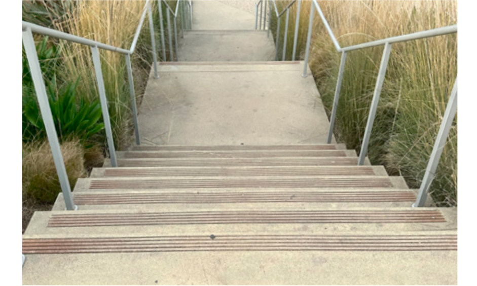
TRACTION GROOVES ON STEPS
