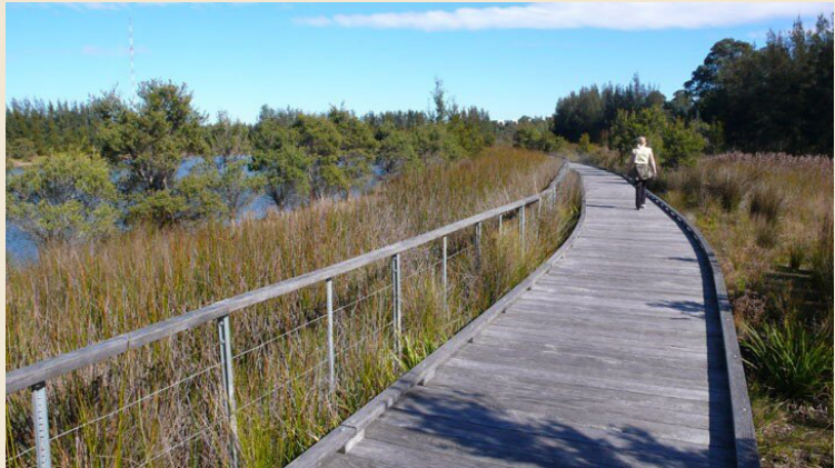
Sydney Olympic Millennium Parklands Sydney, Australia Raised paths through fragile ecological areas
