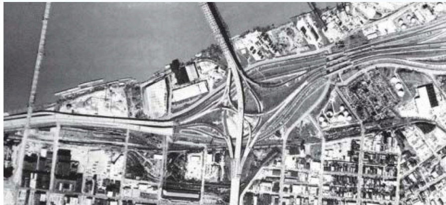
Aerial view of the Louisville Waterfront before construction
