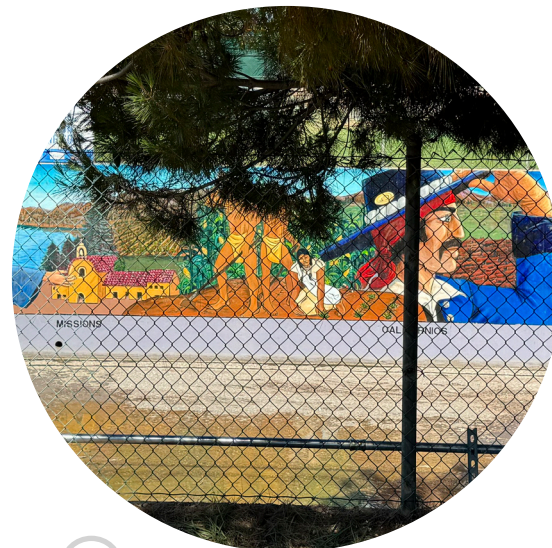
3 Chain link fence around the mural/channel is an eyesore.
