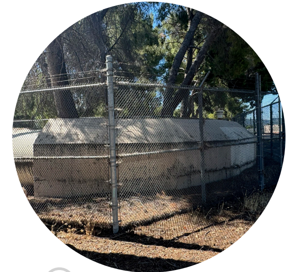
5 Pipe conveyance enclosure on western side of the channel. On the eastern side, the pipe is buried underground, creating an elevation change over the pipe.
