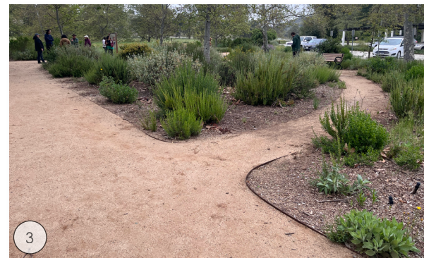
The primary pathway is made of decomposed granite and allows for ADA access and water percolation.
