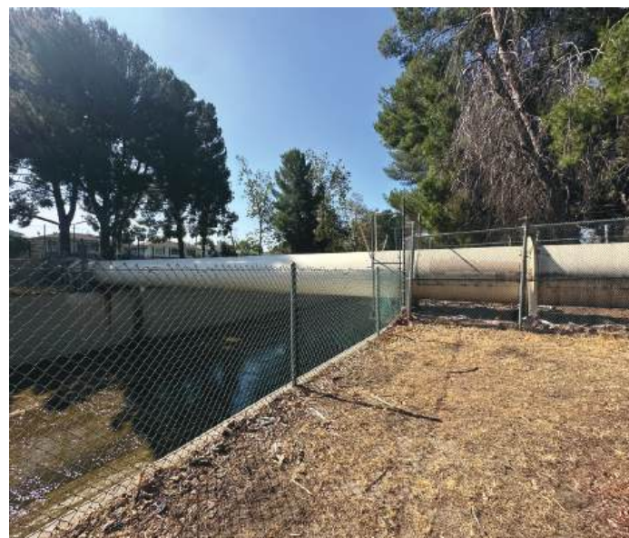
3 LARGE PIPE SPANS CHANNEL
