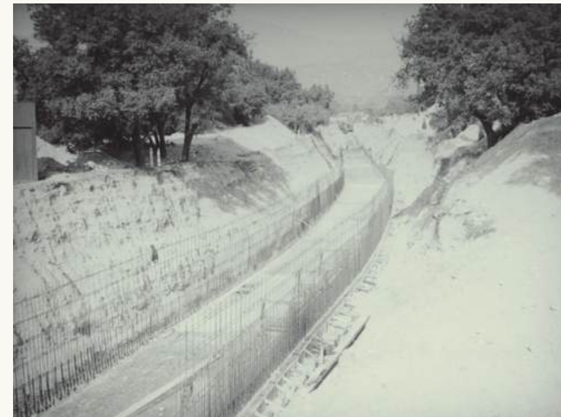
TUJUNGA WASH CONSTRUCTION
