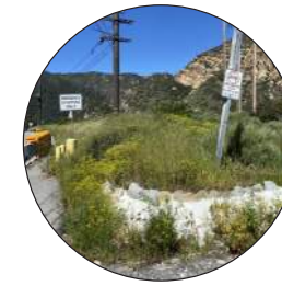
Historical Retaining Wall
