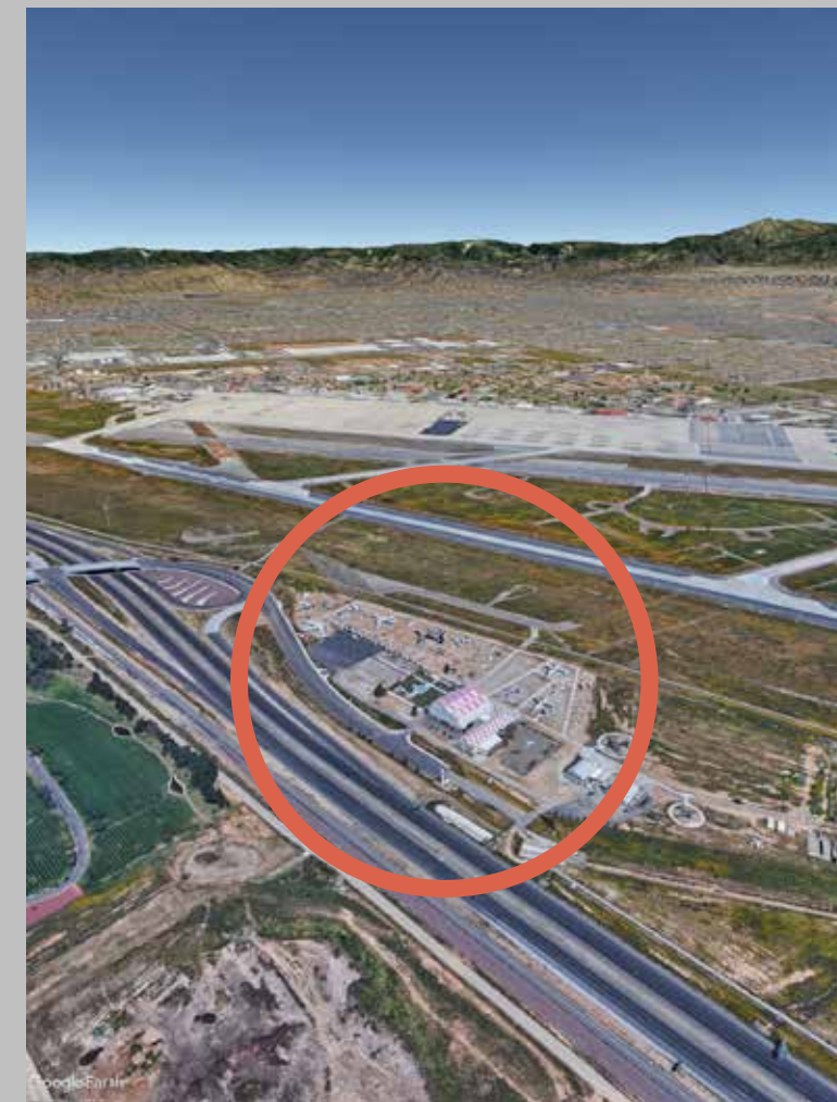
Aerial showing the 215 Freeway, the museum, and the airbase.
