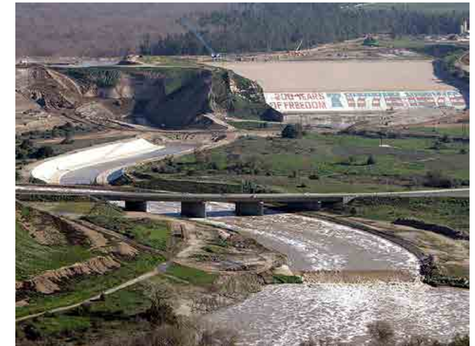
Ensure responsible management and circulation of water on site, recognizing it's important flood management roles.
