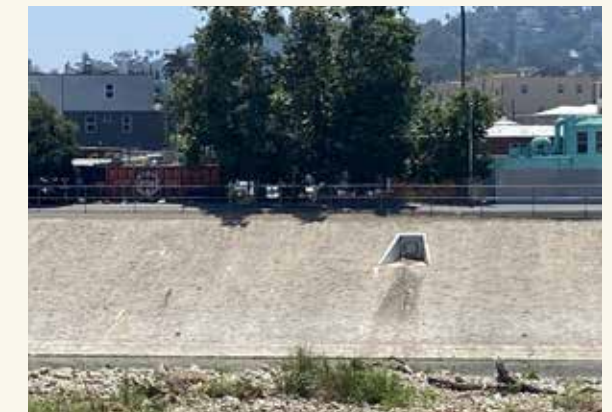
C7 Stormwater Tunnels and Outfalls
