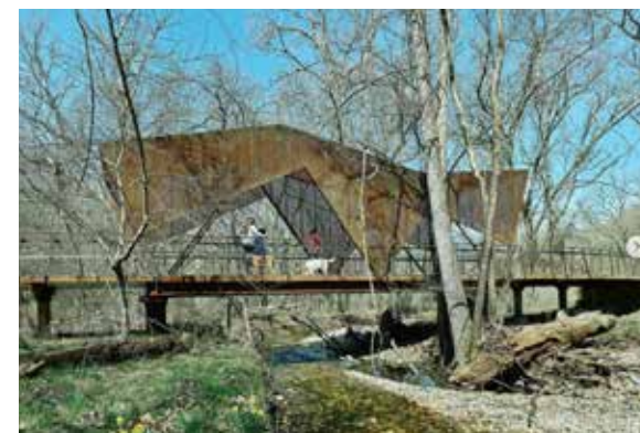
Shaded walkways (elevated over wetlands)
