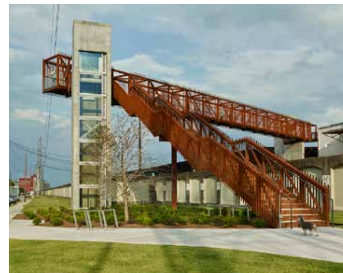
Bridge with stairs and elevator
