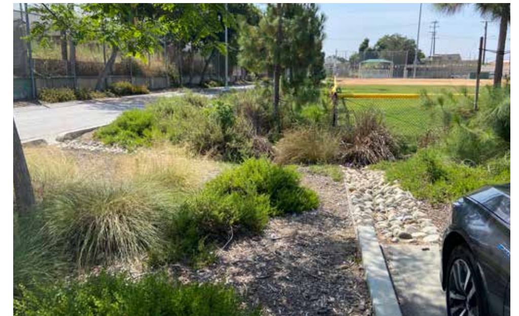
Curb cuts and bioswale
