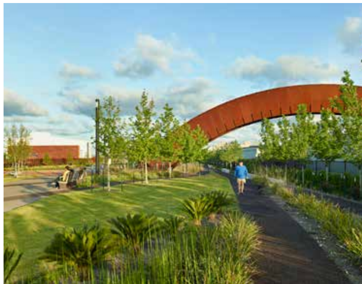
‘Rusty rainbow’ bridge over railroad tracks
